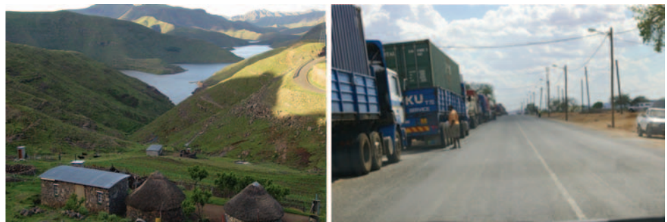
Left: a view of Mohale Dam; Right: trucks backed up waiting to cross the Zambezi River at Tete.
