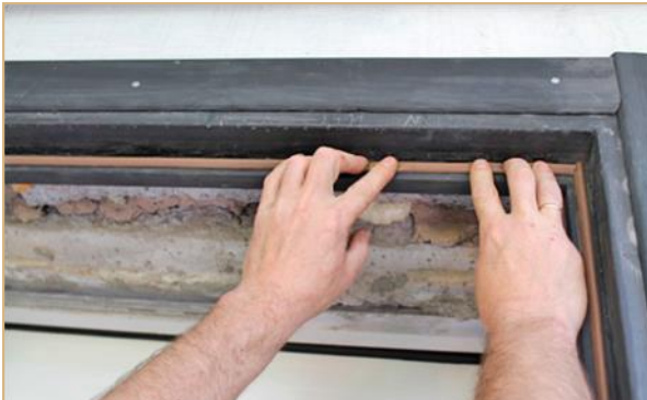
Sealing of doors
