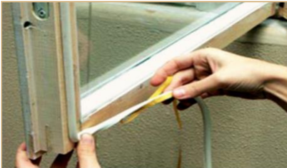
Sealing of window frames
