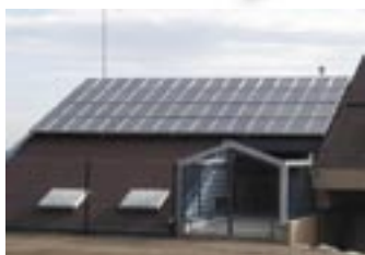
installation photovoltaïque de Saint-Joseph
