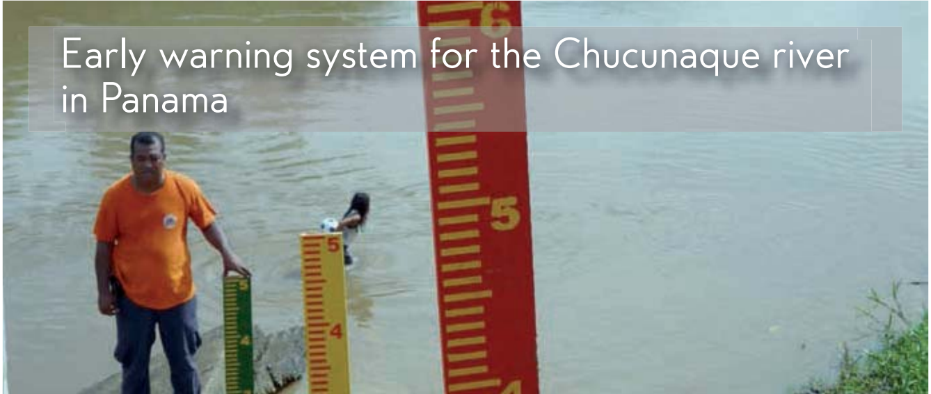
Installation of a limnimetric scale in the Chucunaque River around the El Salto community, Panama
