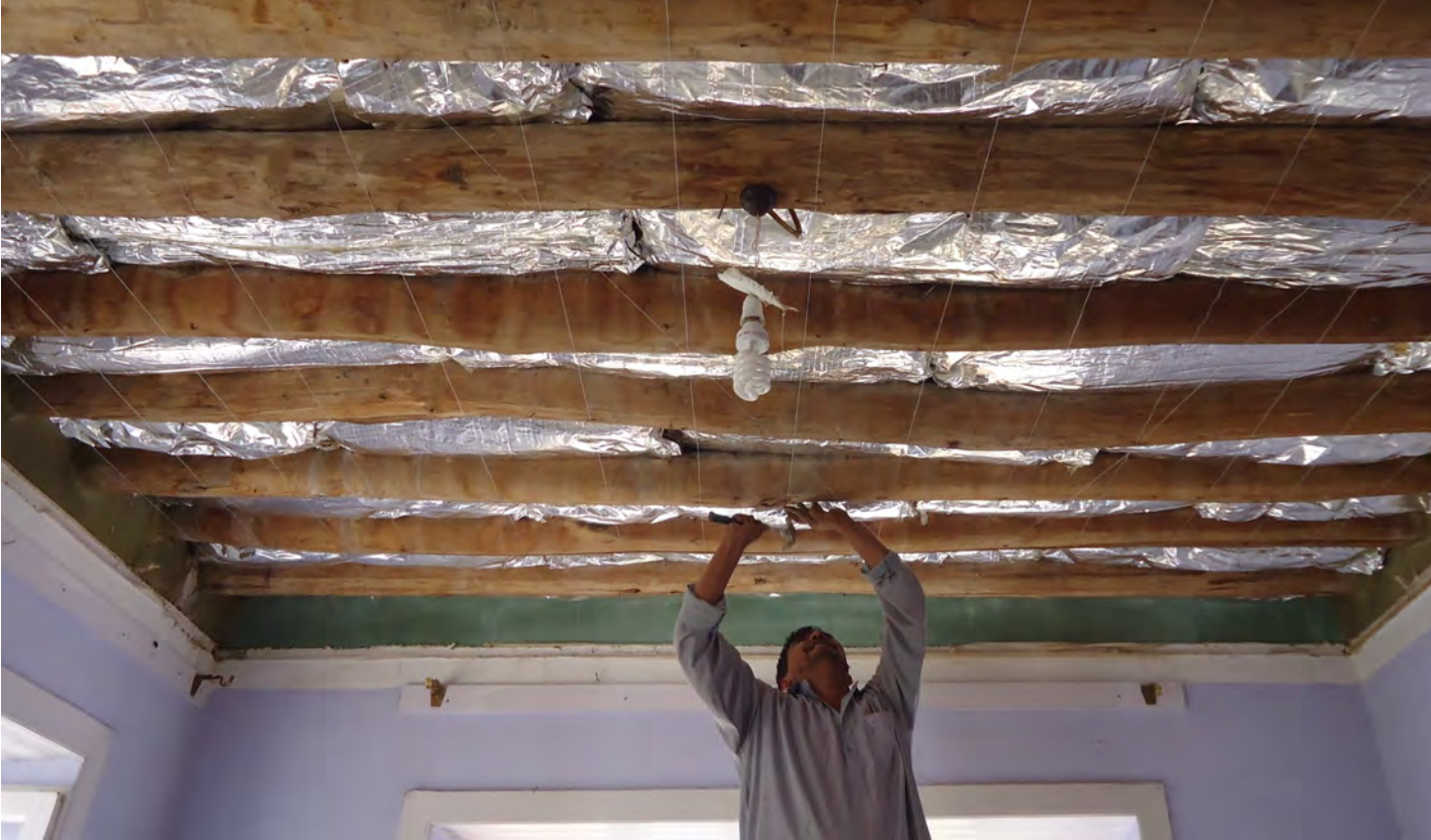
Insulation of the roof using glass wool
