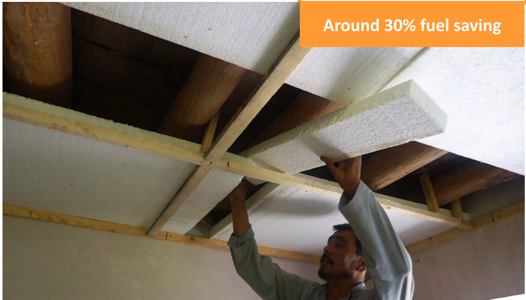
Insulation of the roof using polystyrene
