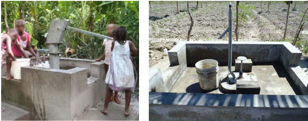
FIGURE 6 : A GAUCHE, POMPE A BRAS (MODELE INDIA MARK) A DROIT, POMPE A PEDALE (MODELE VERGNET HPV-60)
